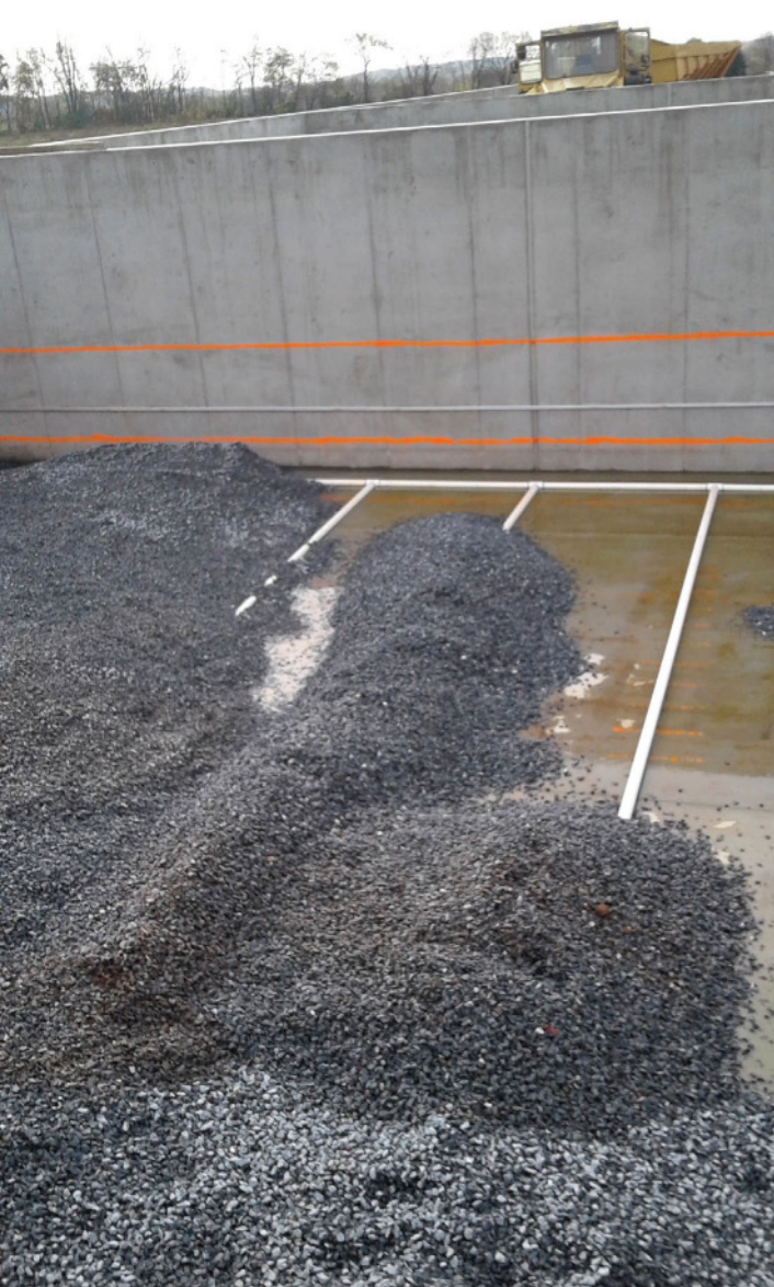
A concrete walled SSF under construction showing PVC pipe drain manifold and larger aggregate to keep sand from clogging drain. The lower orange line is the height of large aggregate, and the higher orange line is the height of filter sand.
