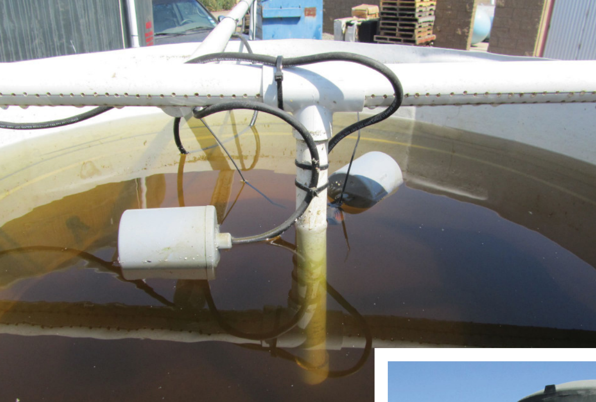
The submerged sand layer of a 40-inch diameter SSF designed to treat runoff from 27,000 square feet of research greenhouses. The float valves control inflow via the PVC manifold when the water level drops. The flow through the sand bed is controlled on the outflow.
