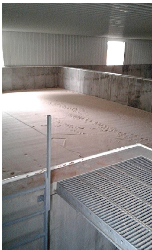
The same concrete walled SSF filter finished before initiating water flow. The PVC pipe around the rim of the concrete is the inflow manifold. As this was in the Mid-Atlantic U.S., a building was built to protect the SSF from freezing.
