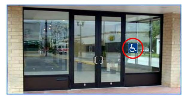
1133B.2.4.1 Thresholds – The floor or landing shall not be more than ½ inch (12.7/mm) lower than the threshold of the door way. Change in level between ¼ inch (6.35 mm) and ½ inch (12.7 mm) shall be beveled with a slope no greater than one unit vertical in 2 units horizontal (50-percent slope). Change in level greater than ½ inch (12.7 mm) shall be accomplished by means of a ramp. See Section 1133B.5.1
