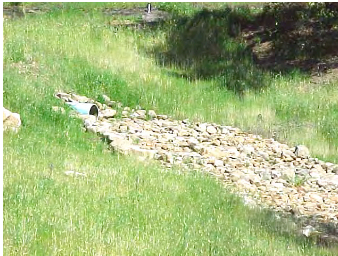
Figure 2. Culvert draining into a rock dissipater
