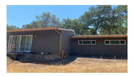
Building 308 is a residential structure referenced as the dormitory located on the east side of the Sierra Foothill Research & Extension Center campus, totaling 1,536 square feet. There are drywall systems within the building, along with multiple vinyl flooring systems. The exterior walls are comprised of wood panels with a shingle and felt roof.
