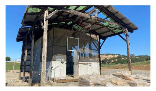
Building 211 is referenced as the cold storage facility and totals approximately 1,200 gross square feet. The building consists of wood beams and metal siding, with a pitched roof with a mix of metal and plastic roof panels.
