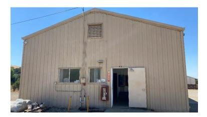
Building 203 is referenced as the feed warehouse, and totals approximately 2,320 gross square feet. The building materials consist of metal roofing and siding, with drywall system and cement floor. The materials sampled in this building include:
