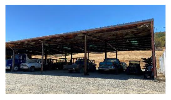
Building 212 is referenced as equipment shed and totals approximately 4,800 gross square feet. The building consists of a free standing metal structure with metal roofing. The materials sampled in this building include:
