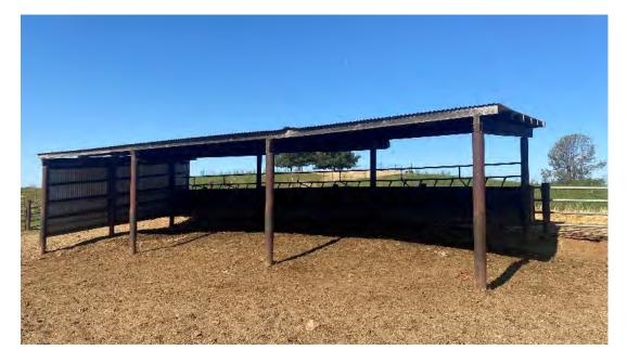
Building 208 is referenced as the bull feeder and totals approximately 320 square feet. The building consists of wood beams and metal roof. The materials sampled in this building include:
