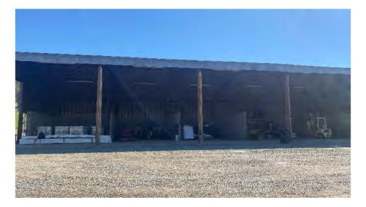
Building 216 is referenced as the bulk feed storage and totals approximately 5,754 gross square feet. The building consists of an open-air metal structure with wood beams and metal roofing. The materials sampled in this building include:
