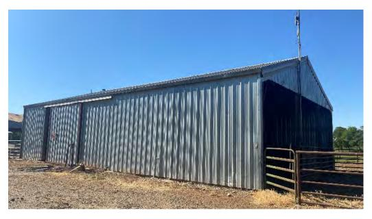
Building 217 is referenced as the calving facility and is the replacement for building 405, artificial insemination building. The building consists of a metal structure with wood beams and metal roofing. The materials sampled in this building include:
