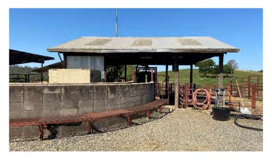
Building 207 is referenced as the scale shed and totals approximately 840 square feet. It is a small open-air structure and consists of wood beams and a metal roof, with concrete flooring. There is also a CMU brick and mortar wall that runs between buildings 207 and 216.
