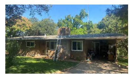
Building 304 is a single-family residence located on the southeast side of the Sierra Foothill Research & Extension Center campus, totaling 1,433 square feet. There are drywall systems within the building, along with multiple vinyl flooring systems. The exterior walls are comprised of wood panels with a shingle and felt roof.
