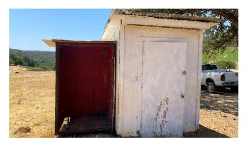
Building 213 is referenced as the pumphouse @ Forbes Headquarters and totals approximately 48 gross square feet. The building consists of a free standing wood structure with metal roofing.
