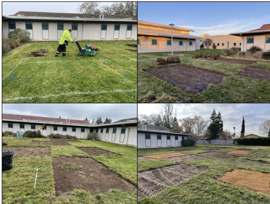
Ongoing work on the turf removal research plots at the Sacramento County Branch Center
