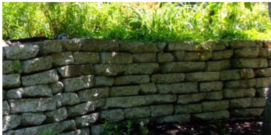
A raised bed constructed from concrete rubble, aka urbanite. Photo: Sharon Gibson.
