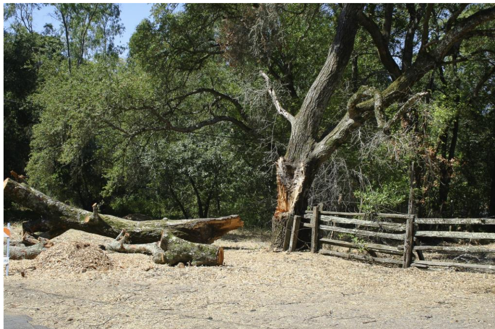
Oak Tree Failure. Photo by Larry Costello, courtesy of the University of California Statewide IPM Program
