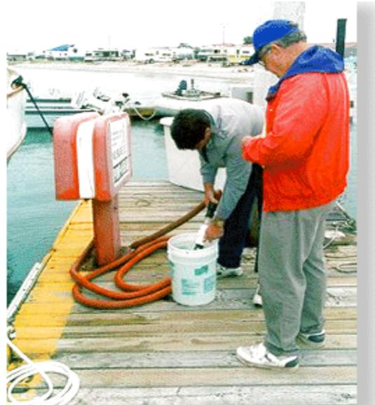
A sewage pumpout station being checked for efficiency. Waste pumped out from boats goes into the local sewage treatment system.
