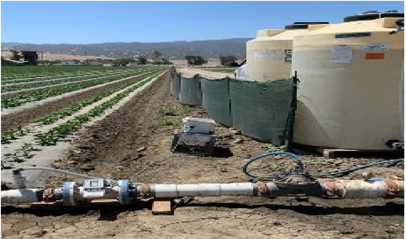
Monitoring irrigation water application and soil moisture levels for efficient irrigation management
