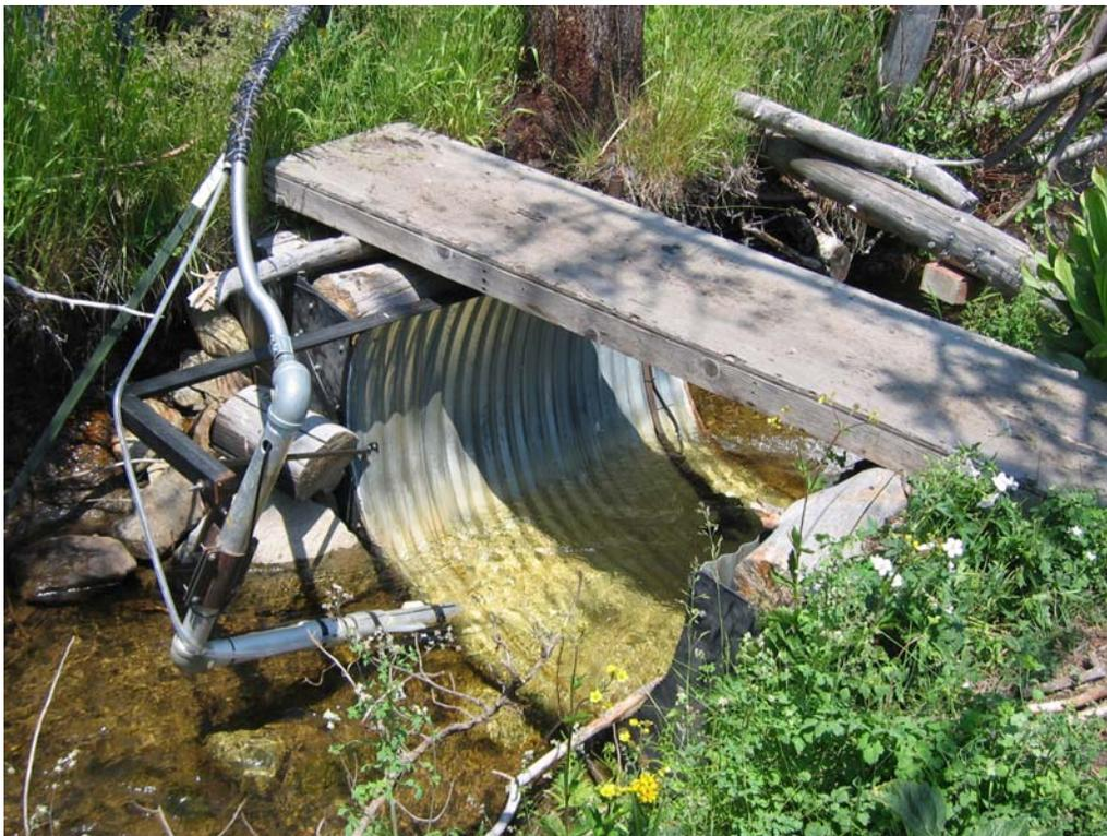
Figure 6. Water quality monitoring station on upper Angora Creek, including boom with recording turbidimeter and a half-round culvert used as a rated section for flow measurement.
