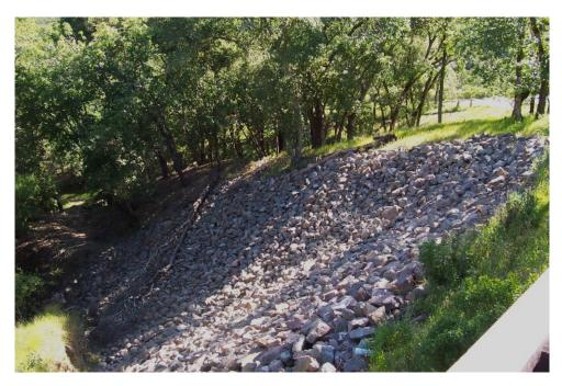
**Figure 12**. Slope protection applied to unstable area along access road, Blue Oaks subdivision, Portola Valley.
