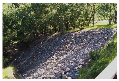
Figure 23. Slope stability enhancement on access road to Blue Oaks subdivision.
