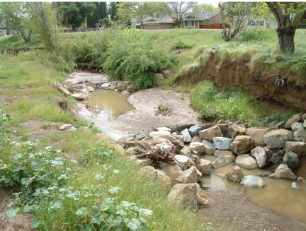
**Figure 6**. Cross vane weirs promoting deposition and channel narrowing, Thompson Creek. This SCVWD project is about three years old (photograph courtesy of J. Owens).
