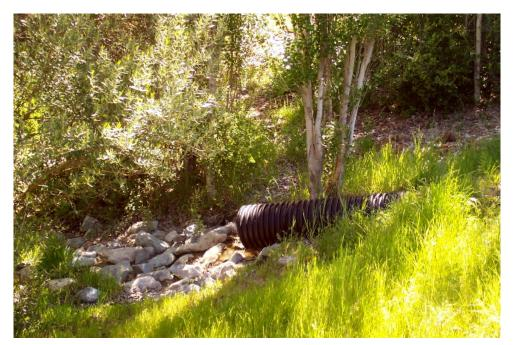
Figure 24. Armored outfall on cross drain, Blue Oaks subdivision.
