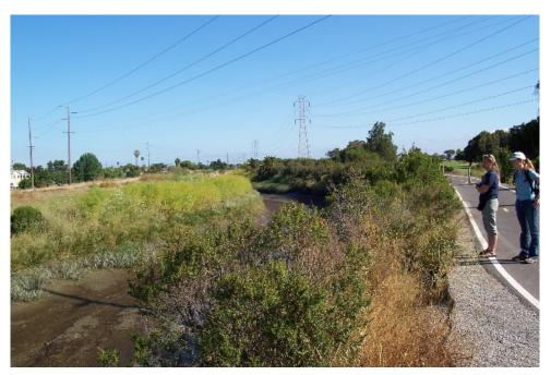
**Figure 14**. Levee on San Francisquito Creek, downstream from Highway 101. Raising the levee had minimal effect on riparian vegetation or instream habitat. Note retaining wall to left of maintenance road that was used to raise the height.
