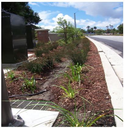
**Figure 16**. Vegetated swale along Sand Hill Road. Road runoff is diverted to the swale through curb cuts (see Figure 17). The swale drains to a catch basin before entering San Francisquito Creek.
