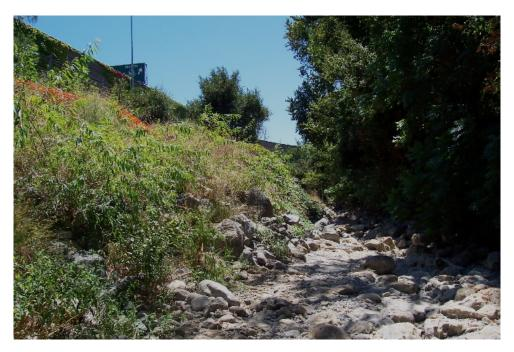
**Figure 7**. Bank stabilization and re-vegetation project applied to failing freeway embankment, Stevens Creek.
