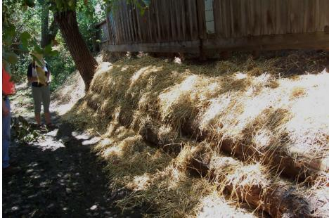
**Figure 8**. Log installation to prevent bank erosion, Permanente Creek. SCVWD uses prescriptive guidelines for all projects involving placement of large wood in streams.
