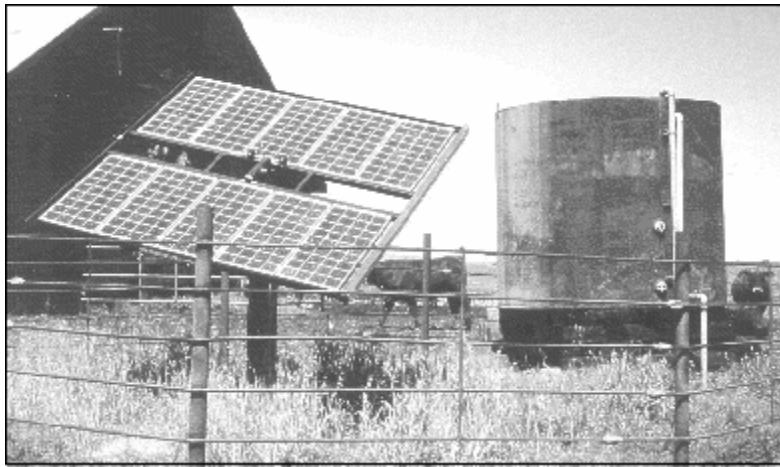
17 gallons a minute with approximately 20 foot of lift. This translates to 1,020 gallons per hour. Water was pumped into a storage tank which then gravity fed into 3 watering troughs. The system was installed to provide an alternative water source to the creek for cattle.
