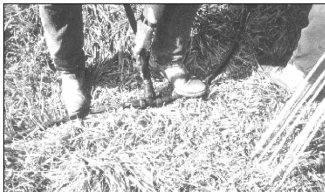
The picture to the left shows how a connection is made. The main line is cut and then each end is inserted through an O ring and then a plastic connector is screwed on. The valve is then upright like a T and is where you insert the pipe.
