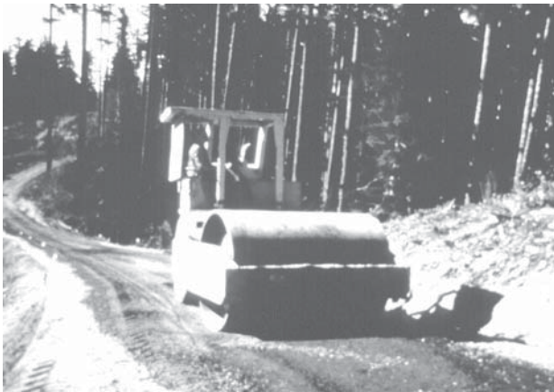
Figure 4-15. Smooth-wheel vibratory roller compacting surface rock.
