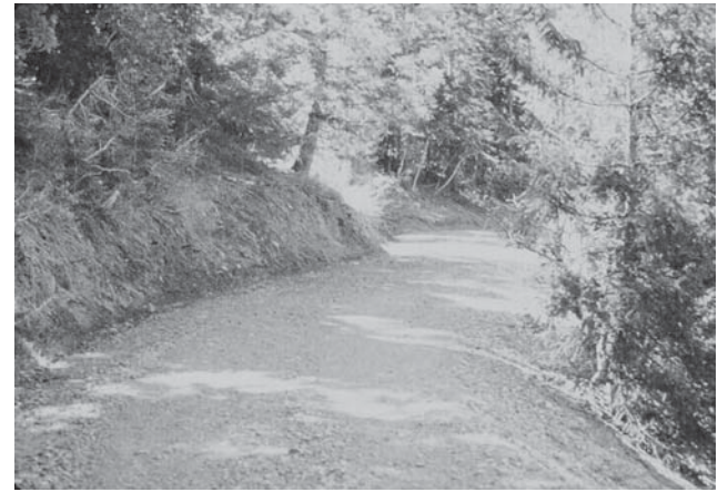
Figure 4-9. Road constructed with well-compacted and -drained subgrade.
