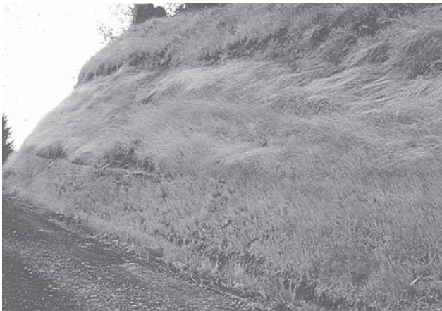
Figure 4-25. Excellent planted grass erosion control on a road cut bank.
