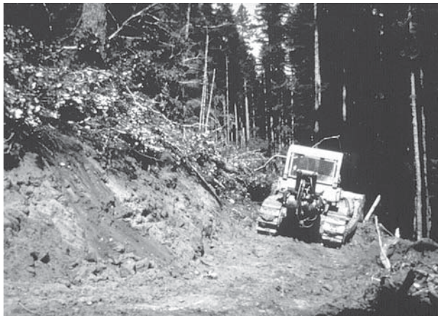
Figure 4-2. Tractor clearing and grubbing.
