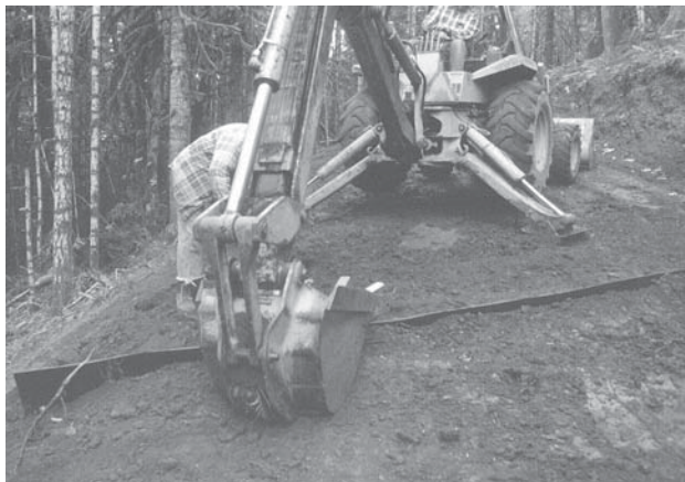
Figure 3-11. Installing a rubber water bar
