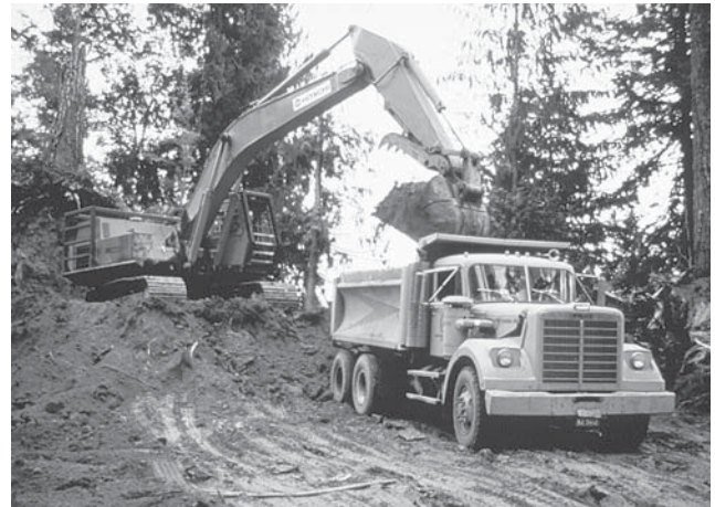
Figure 4-7. Hydraulic excavator excavating roadway material.
