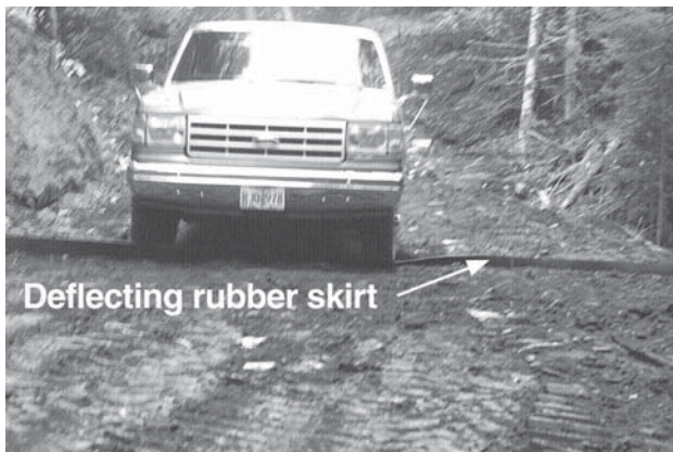
Figure 3-10. A vehicle driving over a newly installed rubber water bar.
