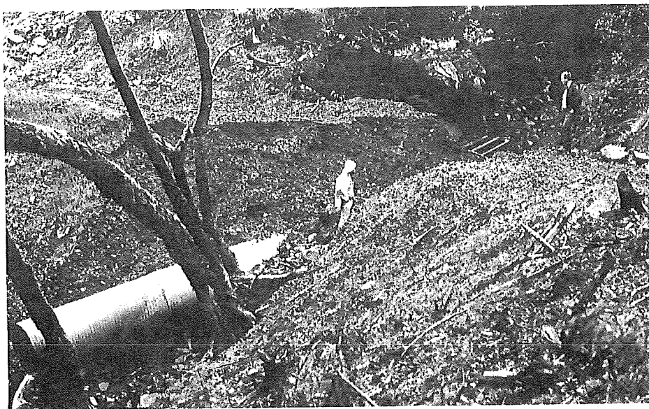
FIGURE 8.4.—Stream crossings pose the greatest risk to fish habitats of any road feature. When culverts are plugged by debris or overtopped by high flows, road damage, channel realignment, and severe sedimentation often result. The capacity of the culvert shown here was exceeded during a heavy storm, and a large slug of sediment was rapidly delivered to fish habitats downstream. Water was not diverted down the road, however. Roads should be constructed so they will not divert streams; where existing roads have the potential to do so, creation of a simple dip or “failure point” will prevent the catastrophic effects that can result from a diversion.
