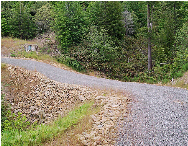
Figure 4. This road has been surfaced with gravel to permit all-season use. Note armoring on stream crossing and dip in the road to prevent diversion of stream flow down the road if the culvert plugs. Photo: Richard Harris.
