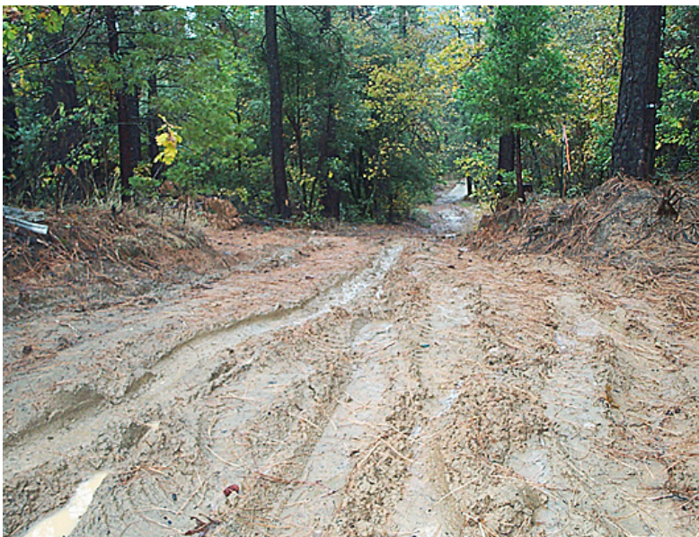
Figure 6. Driving on unsurfaced roads during rainy weather can create ruts and pot-holes that are difficult to repair. Photo: © Angela Wilson; used with permission.
