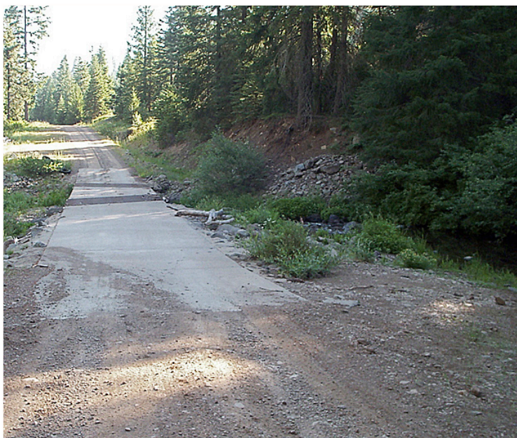
Figure 14. Concrete ford on bedrock outcrop in perennial stream. Photo: © Angela Wilson; used with permission.
