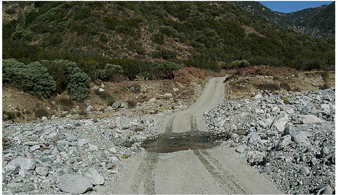
Figure 13. Wet ford stream crossing. These are sometimes called "Arizona crossings." Photo: Richard Harris.
