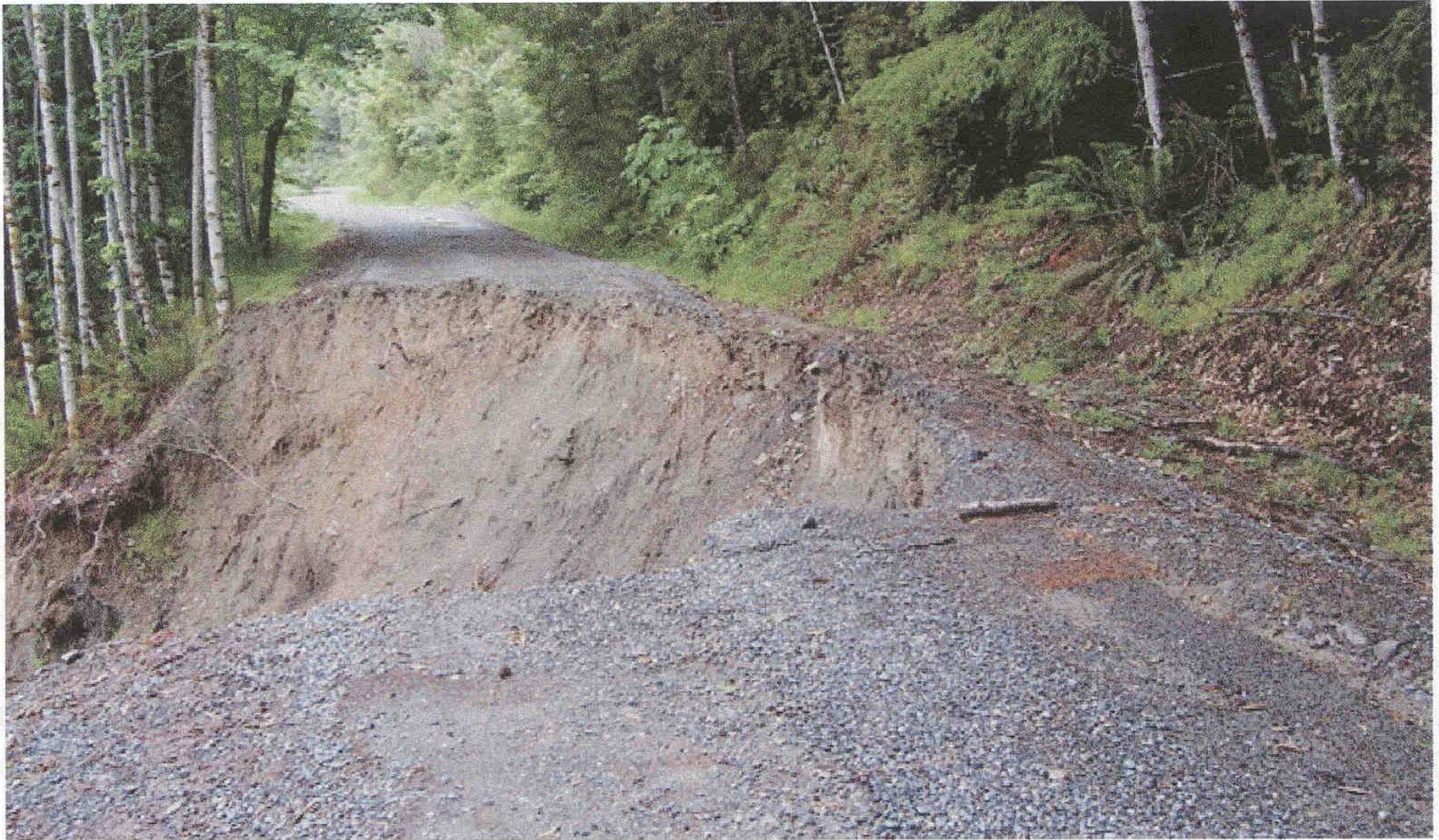
Road failure caused by stream undercutting
