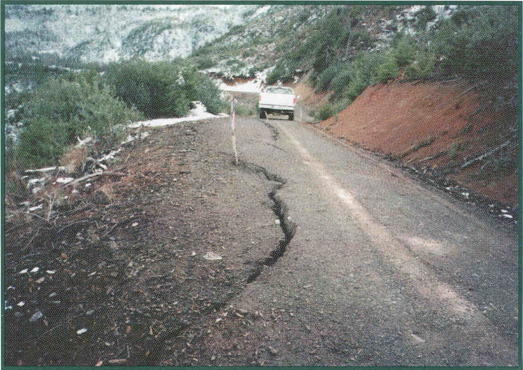
Arc-shaped cracks in sidecast fill are evidence of a landslide starting to move
