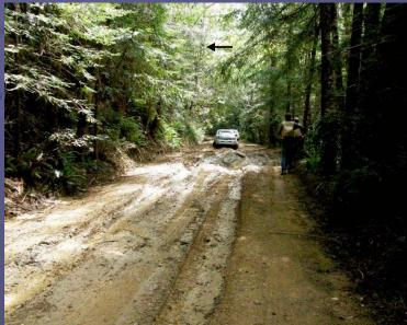
Fill the In Board Ditch, Outslope the Road, Remove the Berm, Breach the Berm, Add Geo Fabric & Rock Surface
