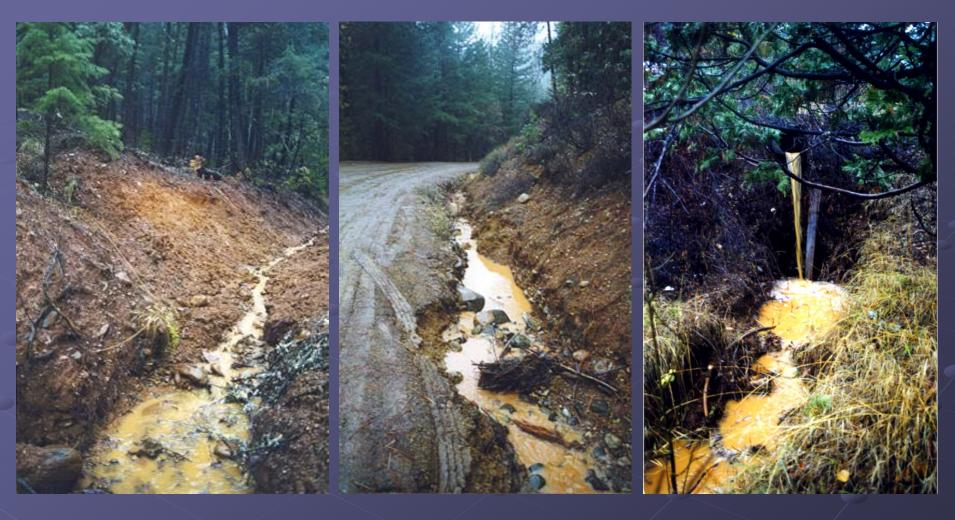
Ditch Activated Erosion Include: Bank Sluff, Bank Slumps, Bank Slides, Bank Surface Erosion, Ditch Downcutting, Ditch Enlargement, Ditch Diversion and Road Cutting
