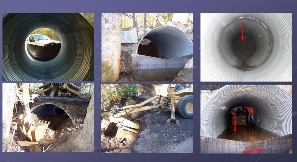
Determine The Proper (D<sub>5</sub>-D<sub>84)</sub> Streambed Mix And Install Using Compaction and Jetting to Seal Fines Within the Larger Gravel/Cobble/Boulder Matrix
