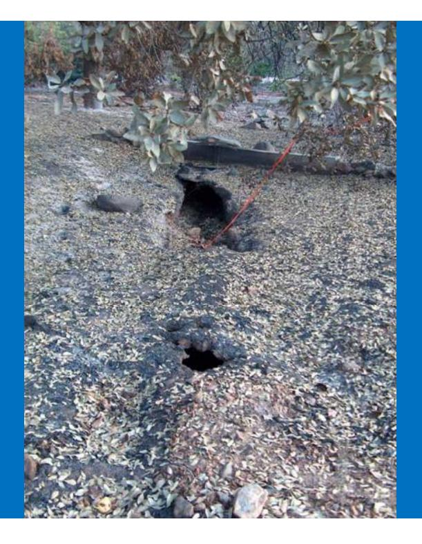
Holes left where plastic culvert burned in small drainages
