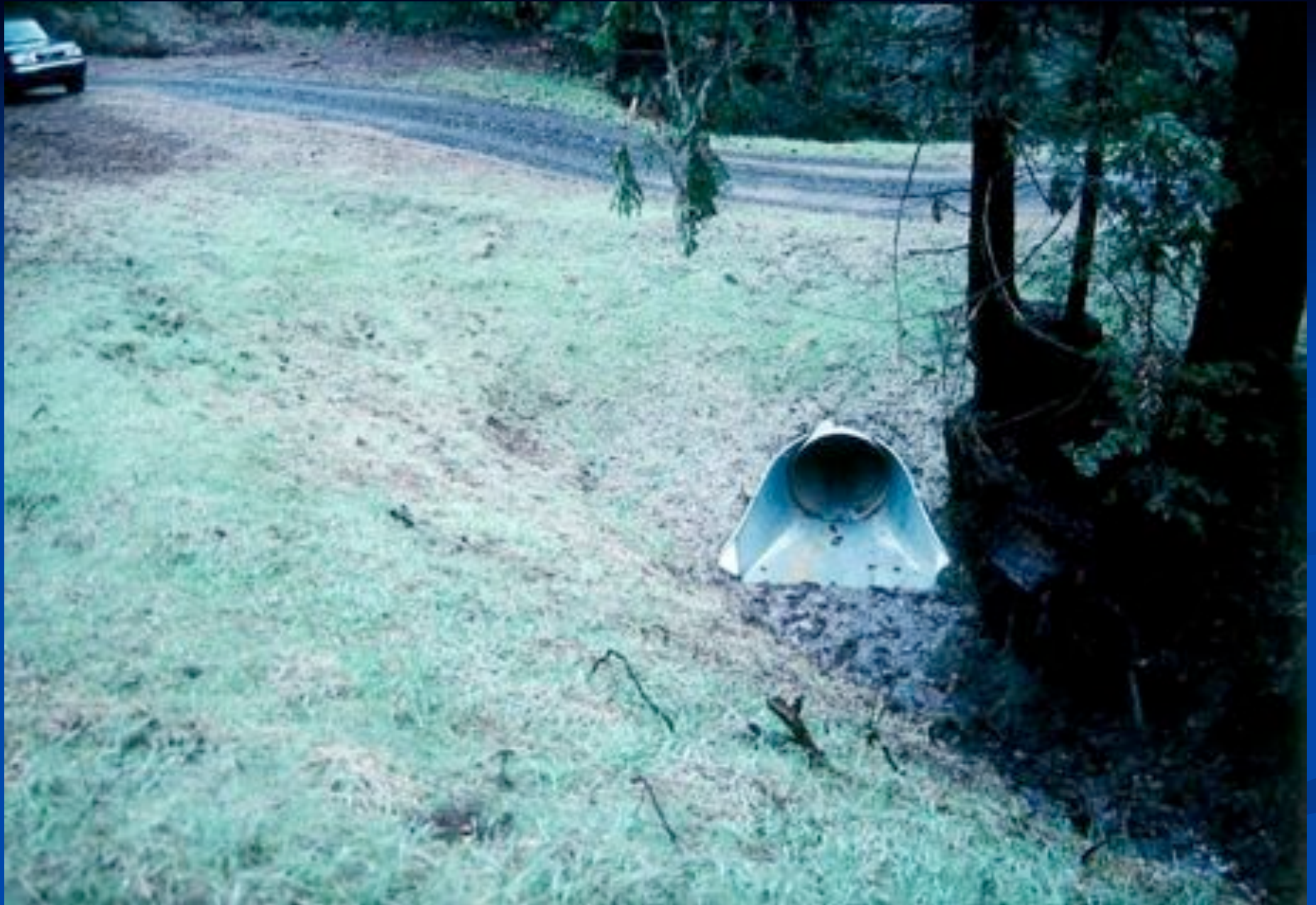
100-yr CMP with flared inlet & critical dip
