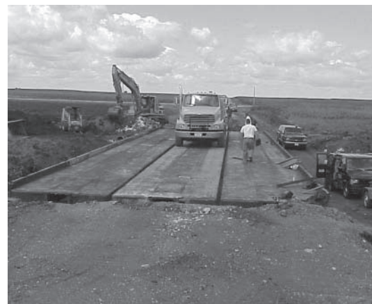
Testing of Winnebago County Bridge before connecting adjacent flatcars.
