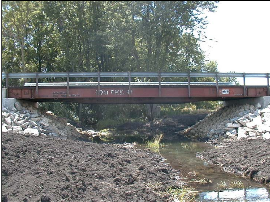
FIGURE 4 Completed 290 th Street Bridge.
