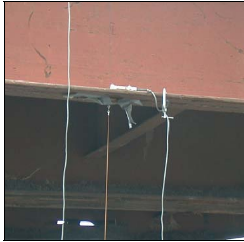
c. Strain transducer on RRFC beam.
