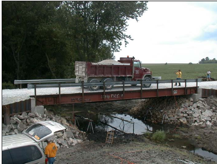
c. Photograph of Test Truck.
