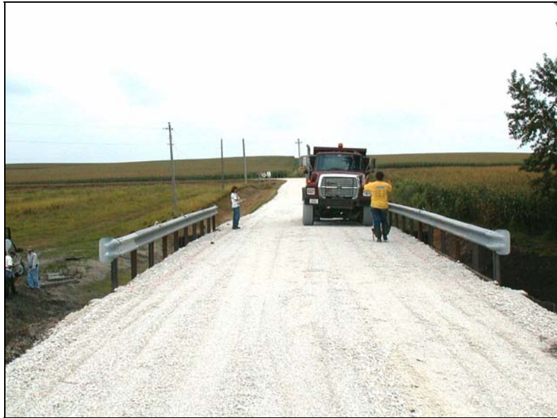
a. Loading bridge with truck on south RRFC (Lane 3).
