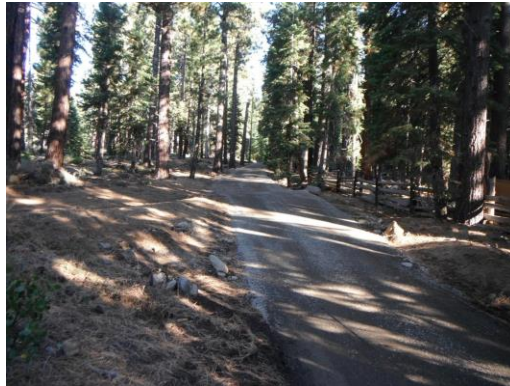
Road drainage improvements on entry road to State Park, Tahoe Basin
