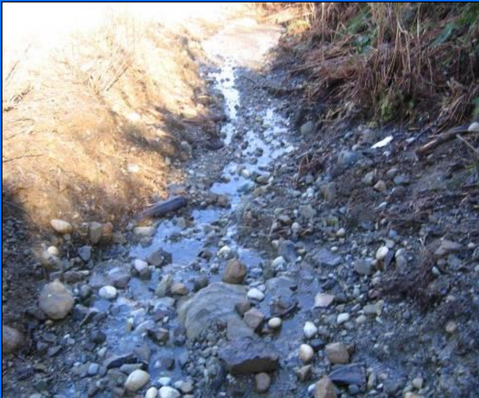
Road ditch with intercepted groundwater
