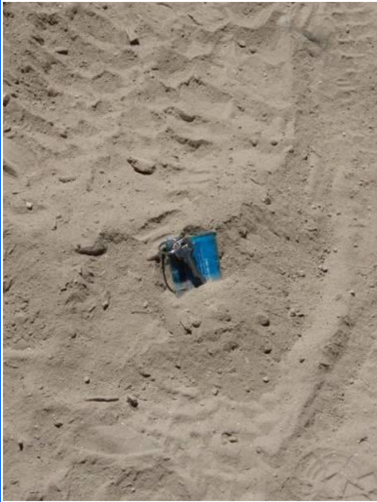
Loose material on road
