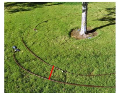
Drip lines with approximate 12" spacing between lines.
