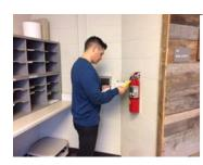
Safety inspections of workplaces and equipment can prevent accidents and injuries at your facility. Cal-OSHA requires scheduled and periodic safety inspections for various equipment and all workplaces. Safety inspections are generally a documented procedure that is conducted by a qualified person using a checklist or form. Cal-OSHA, Title 8, Section 3204 requires records of scheduled and periodic inspections to identify unsafe practices and conditions to be maintained for at least one year.
