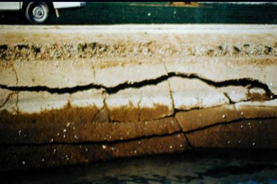
Canal Lining Destruction Due to Piping of Dispersive Soils
