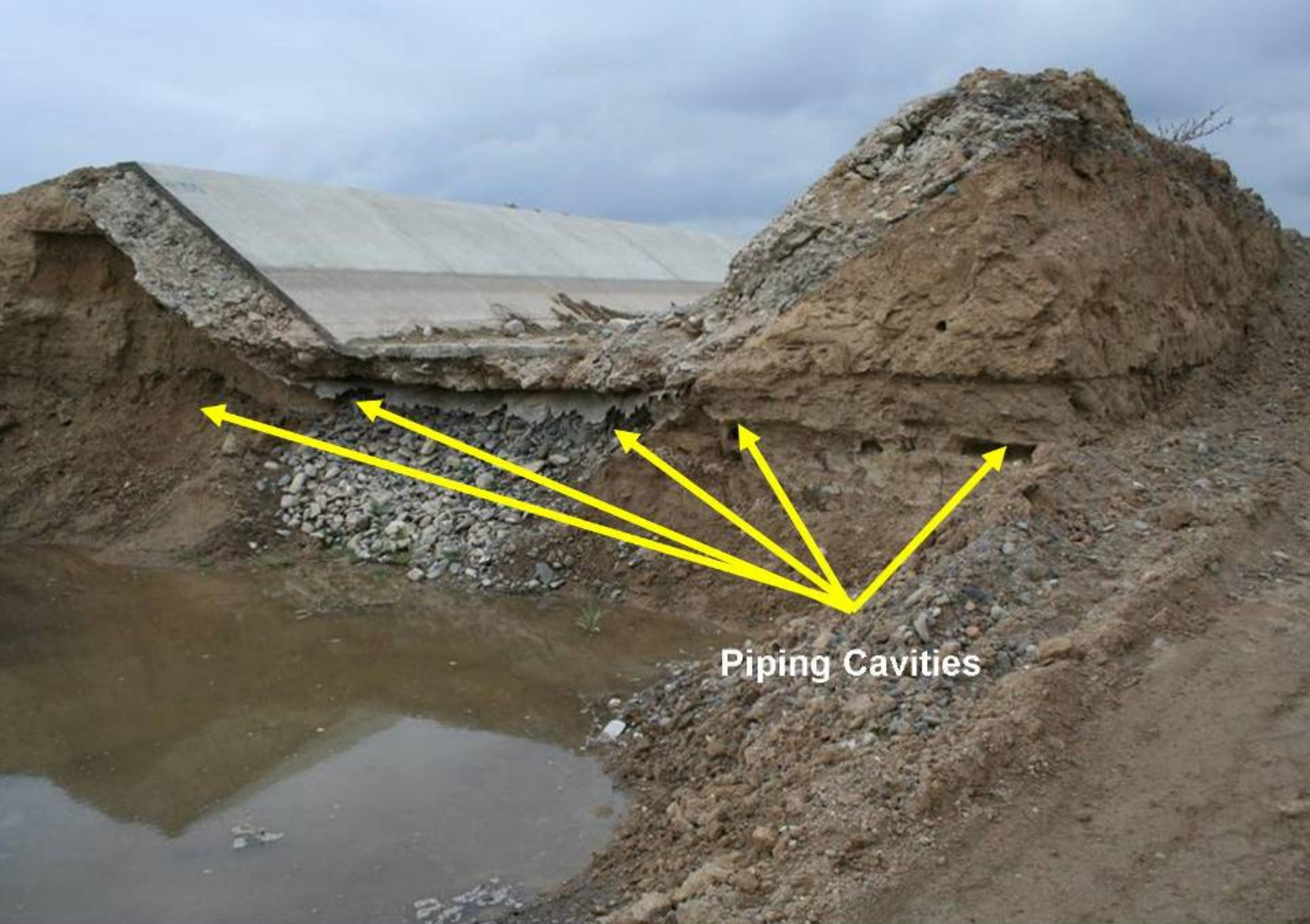
Piping Cavities Under the Old Concrete Lining
