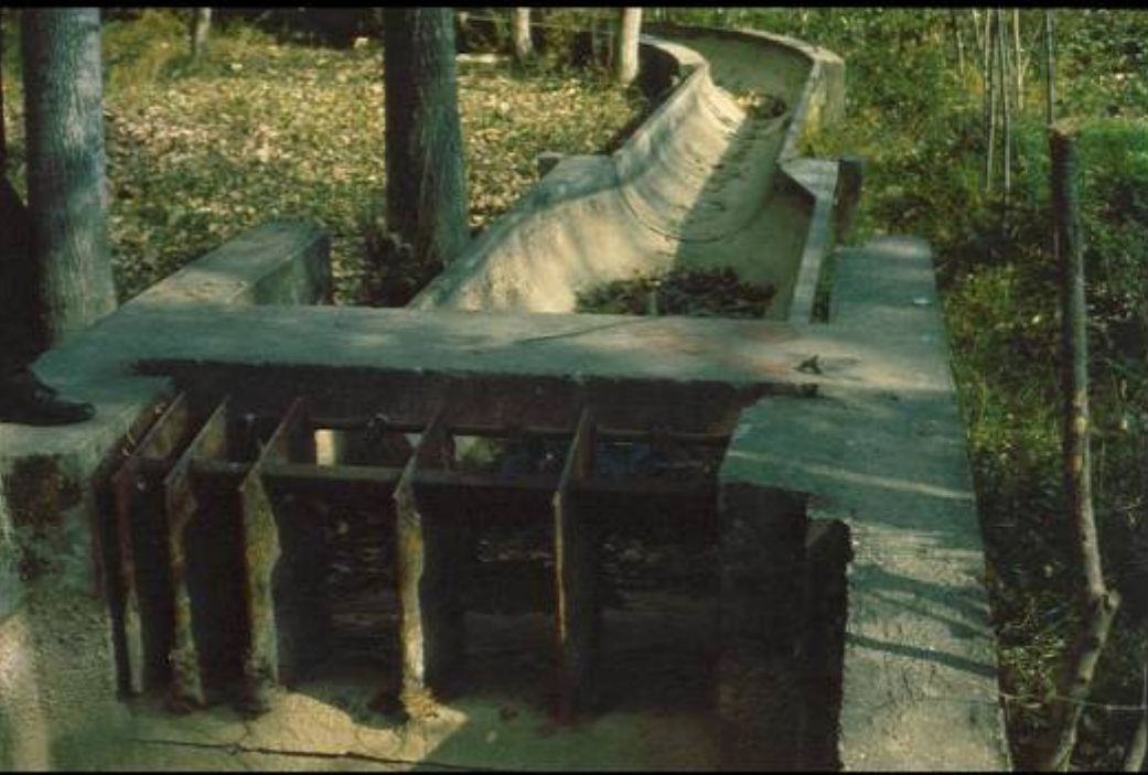
Improper Servicing of the Gates
