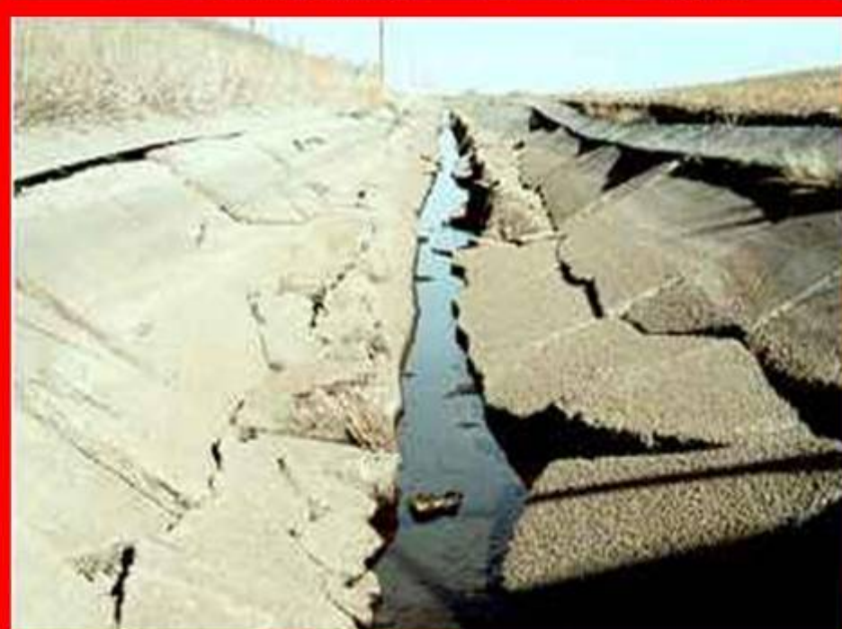
Canal Destruction Due to Unstable Subgrade
