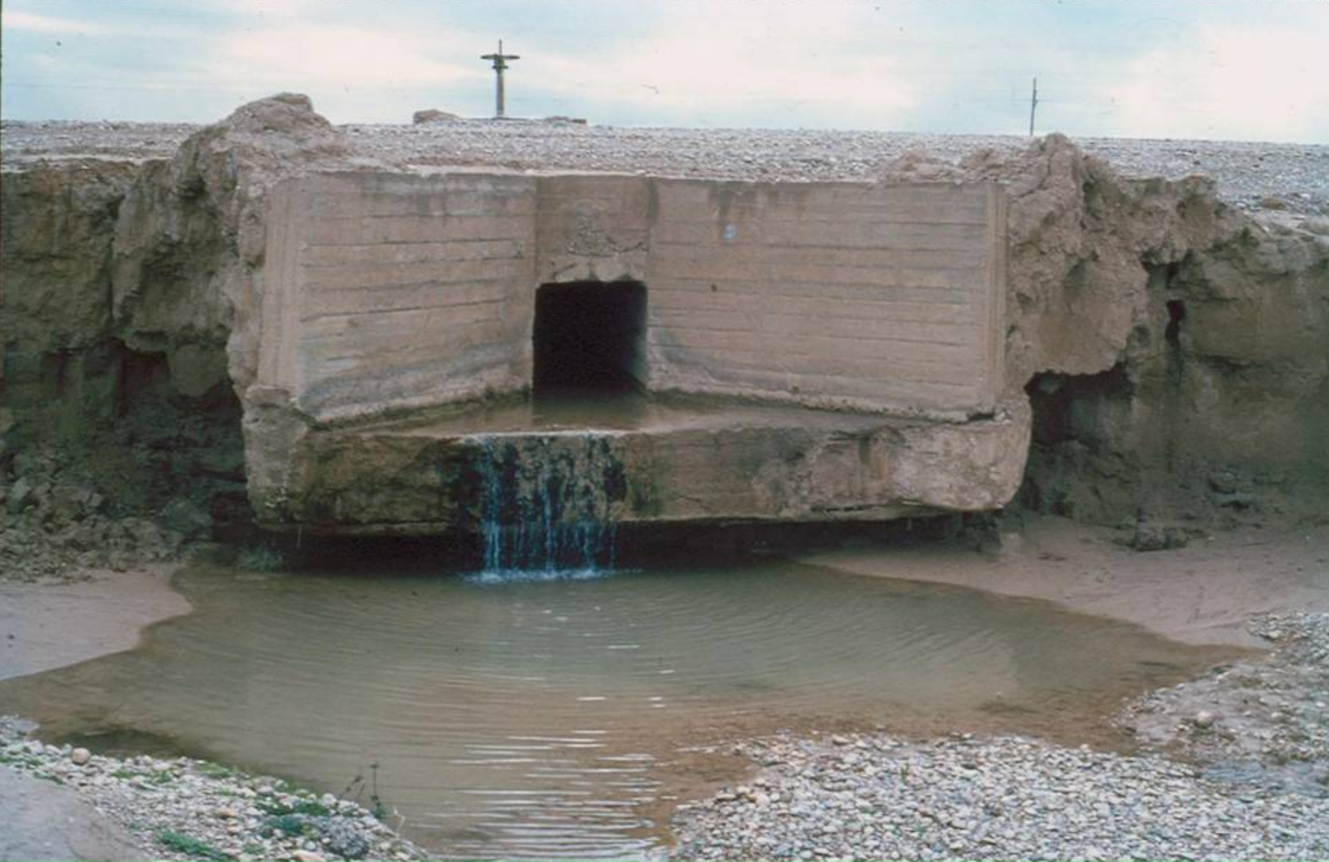
Erosion of Subgrade Soil Due to Presence of Dispersive Soil
