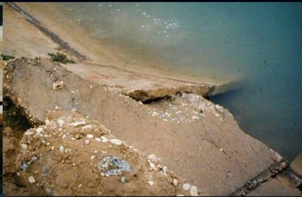
Canal Lining Destruction Due to Piping of Dispersive Soils
