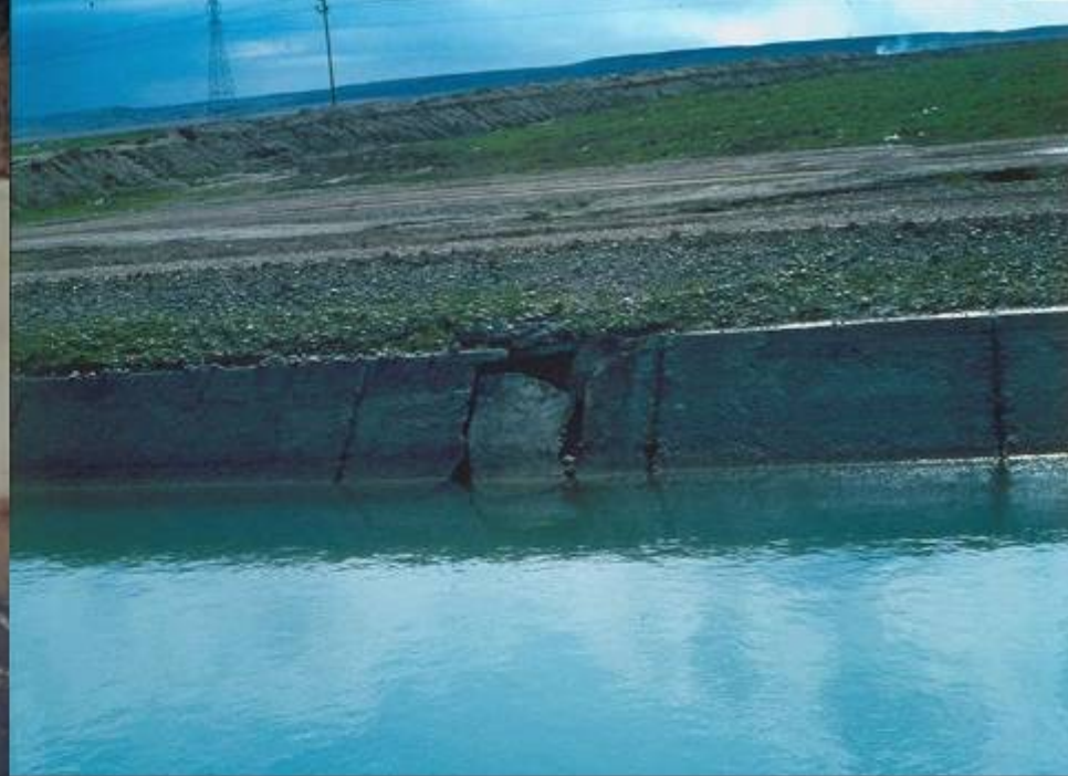
Canal Lining Destruction Due to Piping of Dispersive Soils
