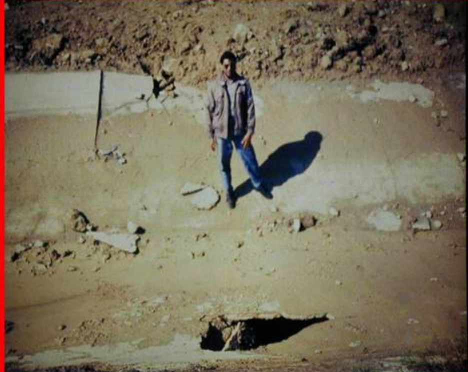
Cavities Under Concrete Lining Due to Solution of Gypsum
