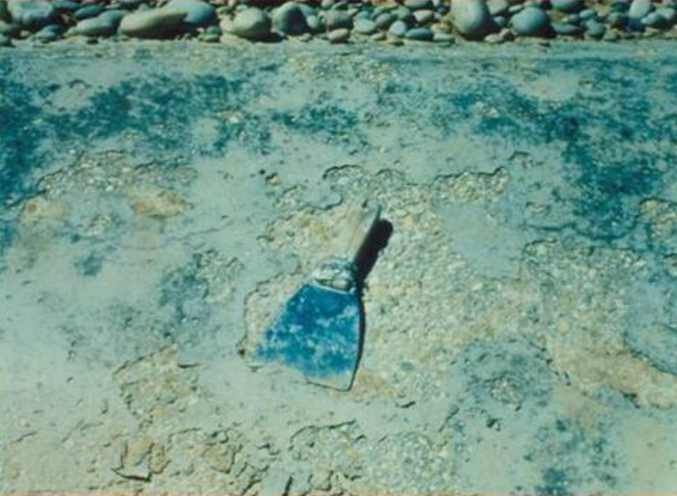
Damages to the Canal Lining Due to Low Quality Concrete
