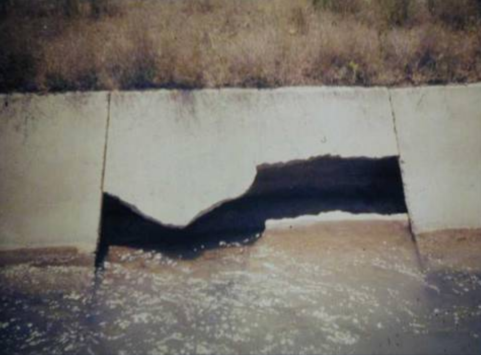
Canal Lining Destruction Due to Piping of Dispersive Soils
