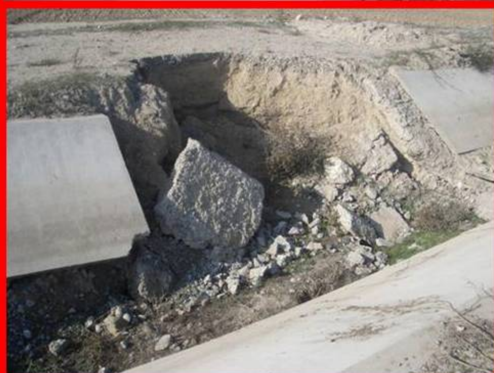
Formation of Cavities Under Canal Lining
