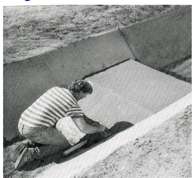
Long-throated flumes that measure channel discharges with minimum head loss are most economical, perform with high accuracy and do not
