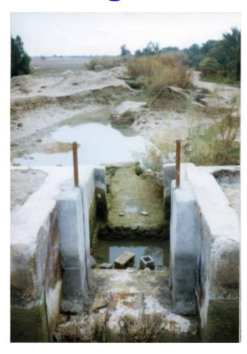
Unfortunately, farmers alter proper functioning of upstream structures used for controlling water level. The Amil regulator used for automatic control of upstream water level (Sarghanat channel network), is no longer functional due to placement of stones and metal pieces by the farmers.
