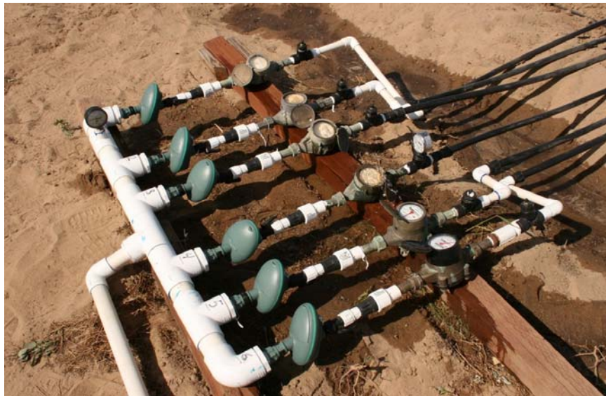
Figure 2. Irrigation control manifold.
