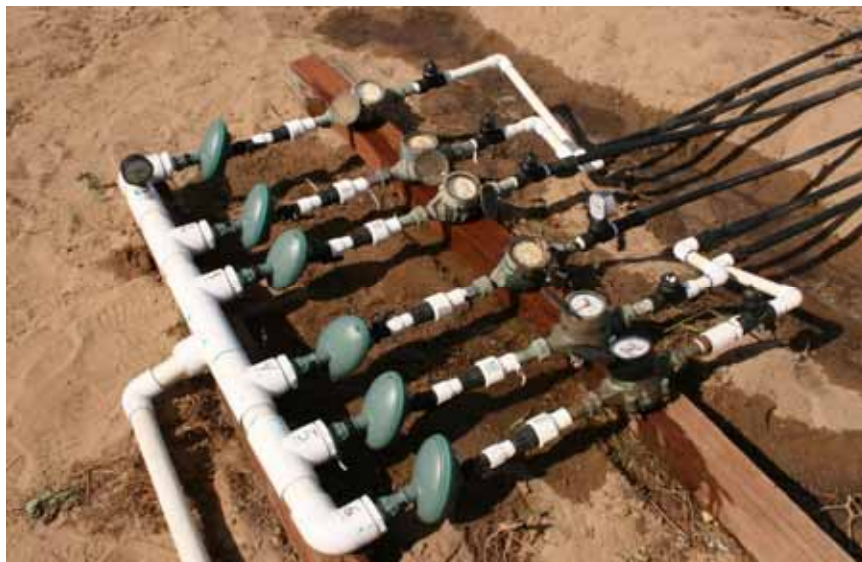
Figure 2. Irrigation control manifold.
