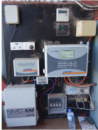
FIGURE 1.9 Automated microirrigation controls. Photo courtesy of Blake McCullough-Sanden, University of California.
