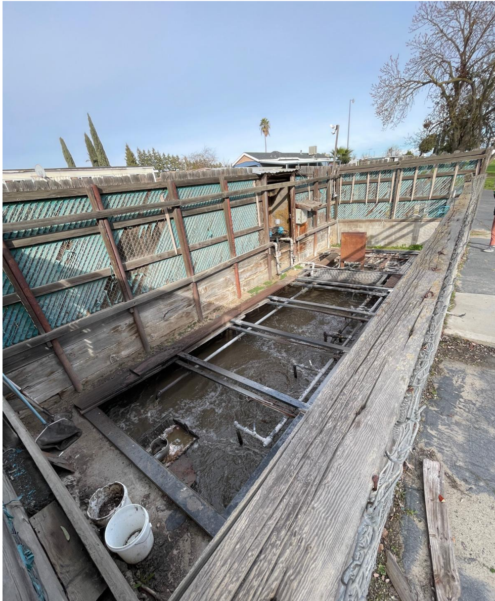
An aeration tank (or extended aeration basin) from the Comunidad Nuevo Lago Mobile Home Park. Photo credit: California Institute of Water Resources
