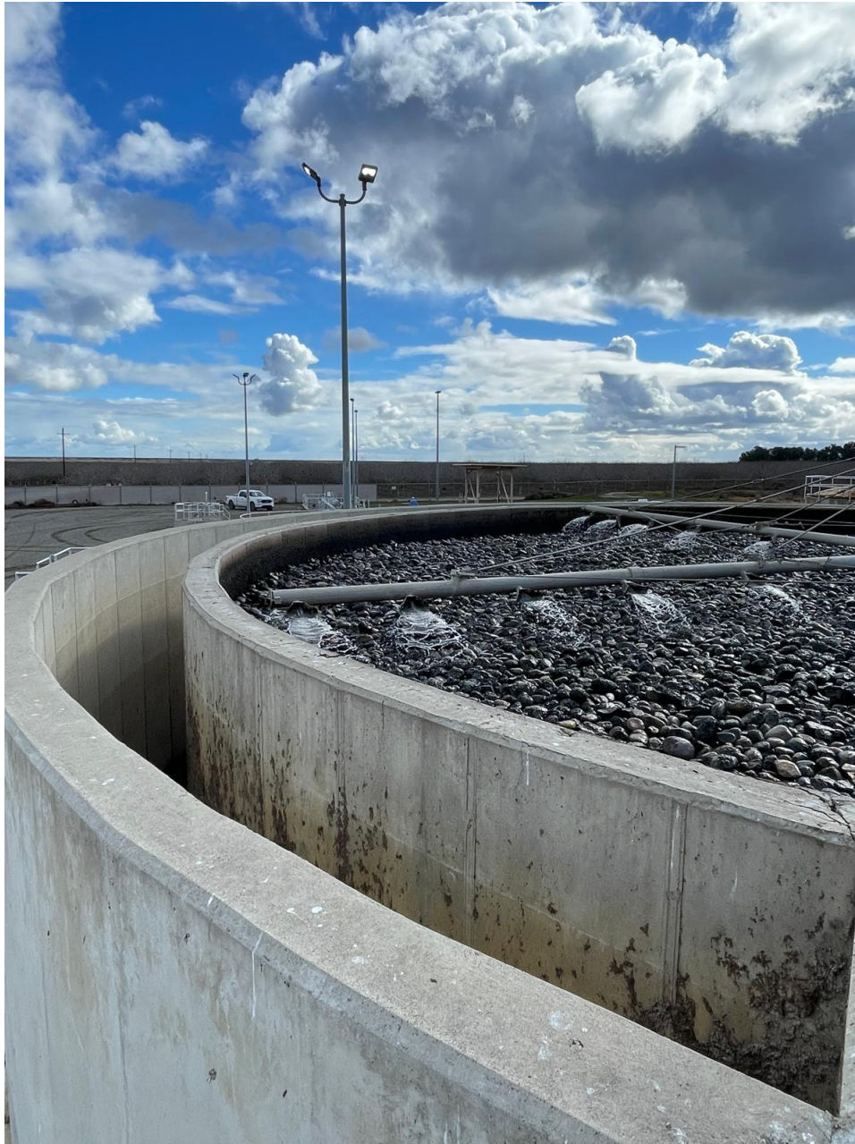
A trickling filter is used as one of the biological treatment stages at the Kettleman City wastewater treatment plant. Photo credit: California Institute of Water Resources
