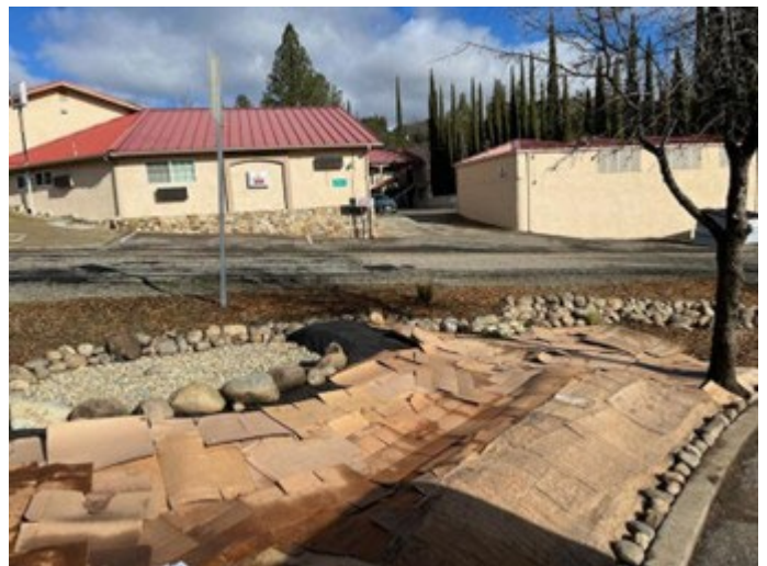
Figure 7 Berms and swales to slow and spread water, reducing flooding.
