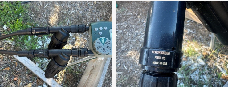
Figure 2. The controller, filters and pressure regulators (left) and detail of one pressure regulator (right)
