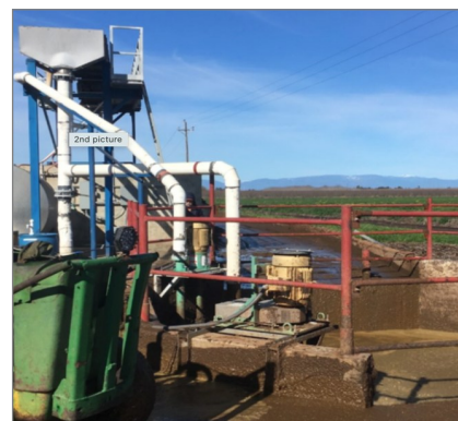
Solid separator and manure storage
