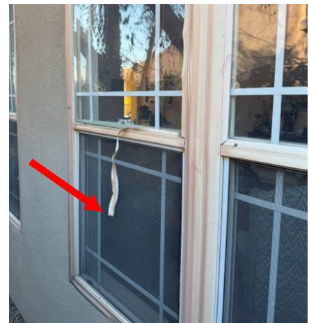
Figure 6: Radiant heat damaged this window. Note the vinyl glazing is deformed. In some cases, radiant heat led to window panes breaking or falling from the frame.
