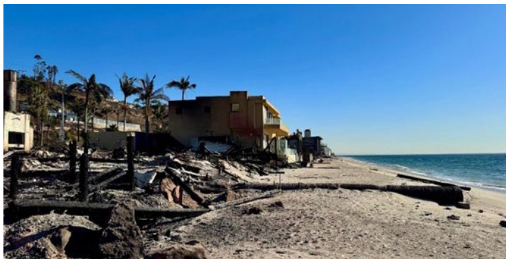
Figure 2: The Palisades Fire burned to the beach, taking many homes along the coast in its path. Some of the surviving buildings illustrated effective home hardening, such as having dual-paned tempered glass windows.
