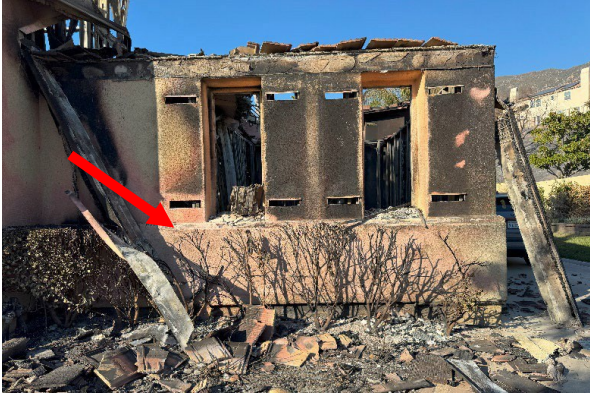
Figure 3: These woody shrubs likely contributed to the radiant heat damage that broke the window in this home. Implementing a 5-foot noncombustible perimeter (Zone 0) is best practice.
