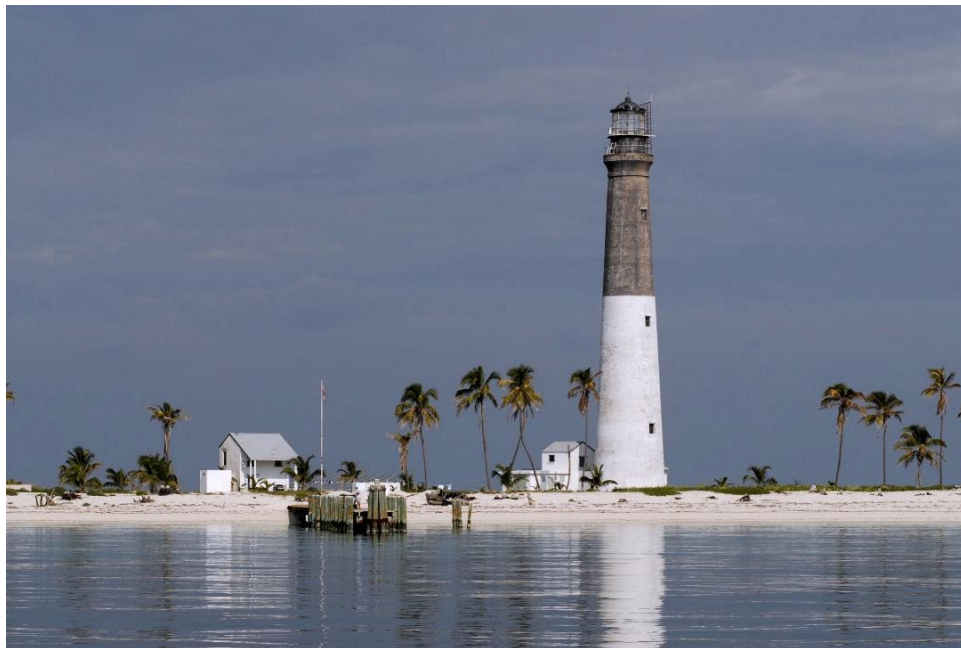
7. Dry Tortugas National Park. Loggerhead Lighthouse. Coconut palms have naturalized on the island. Source: photo credit U. S. Coast Guard, 2005, Jennifer Johnson.
