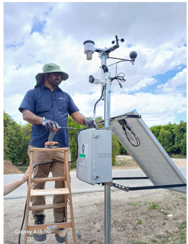
Installation of weather monitoring station at Bardsdale Ranch. Photo: K Bharambe
