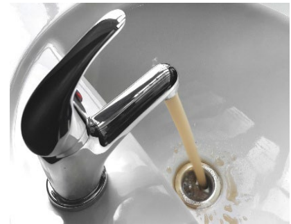
Figure 2: Contaminated water from a faucet. PC: CDC Environmental Health Services
