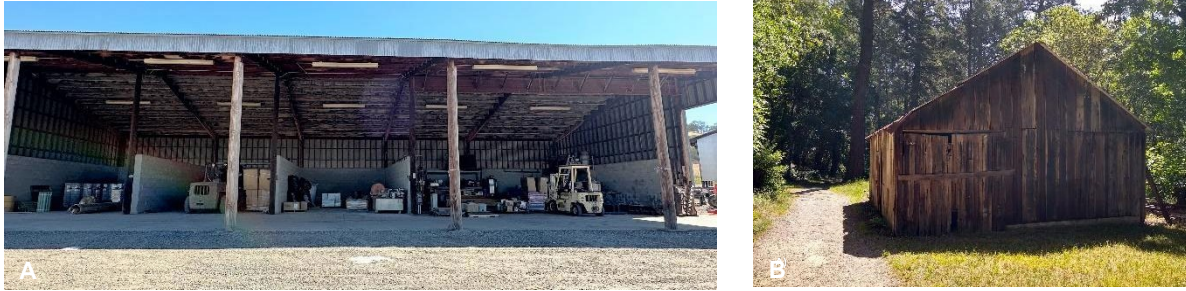
Figure 3: A) Pole barn used to store equipment and materials and B) Enclosed wooden barn surrounded by vegetation.
