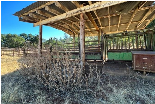
Figure 8: Remove and dispose of vegetation that collects around the first 5 feet of structures.
