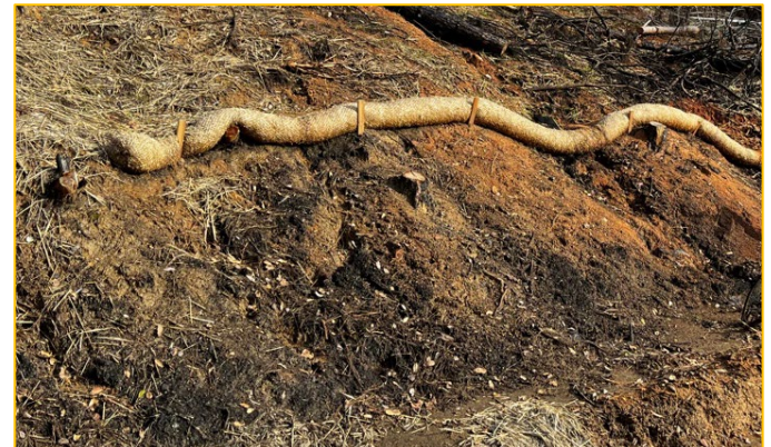
Image 2. A failed erosion barrier that led to channelized flow during a high-intensity rain event [Credit: Alison Deak]
