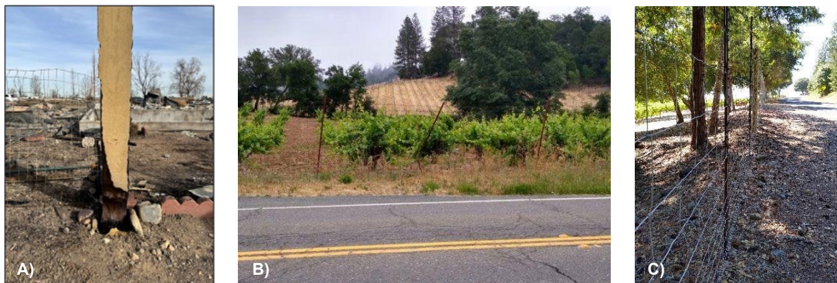
Figure 12: A) Fence post that was burned but fire did not carry due to metal fencing material. B) Metal fence but line not maintained and kept clear of vegetation that can easily carry fire. C) Metal and wooden fence clear of vegetation and well maintained.
