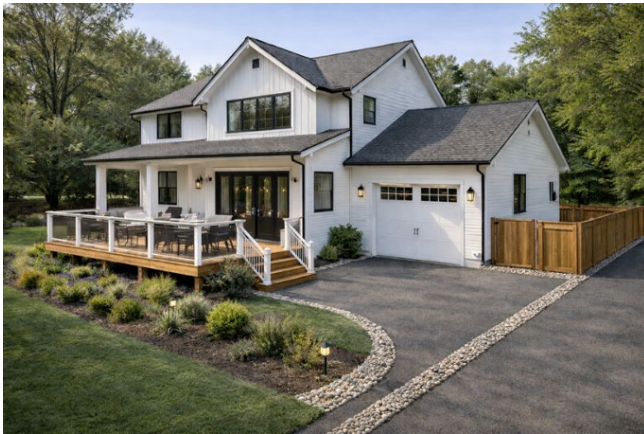
Figure 6. Before-and-after representation of a single-family house that implemented Zone 0. Note the relocation of the plants away from the deck and the installation of a noncombustible gate. While not required, it is best practice to install metal screening around the deck base to keep embers and debris out. Once Zone 0 is finalized, the guidance document will provide tips for addressing issues like this.
