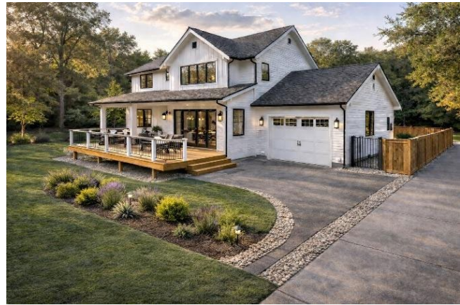
Figure 6. Before-and-after representation of a single-family house that implemented Zone 0. Note the relocation of the plants away from the deck and the installation of a noncombustible gate. While not required, it is best practice to install metal screening around the deck base to keep embers and debris out. Once Zone 0 is finalized, the guidance document will provide tips for addressing issues like this.
