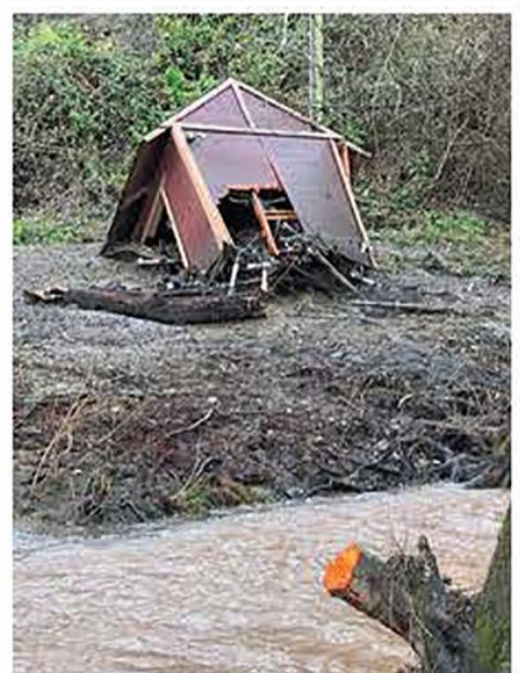
The storm knocked down the water pump house and the equipment was washed away.
