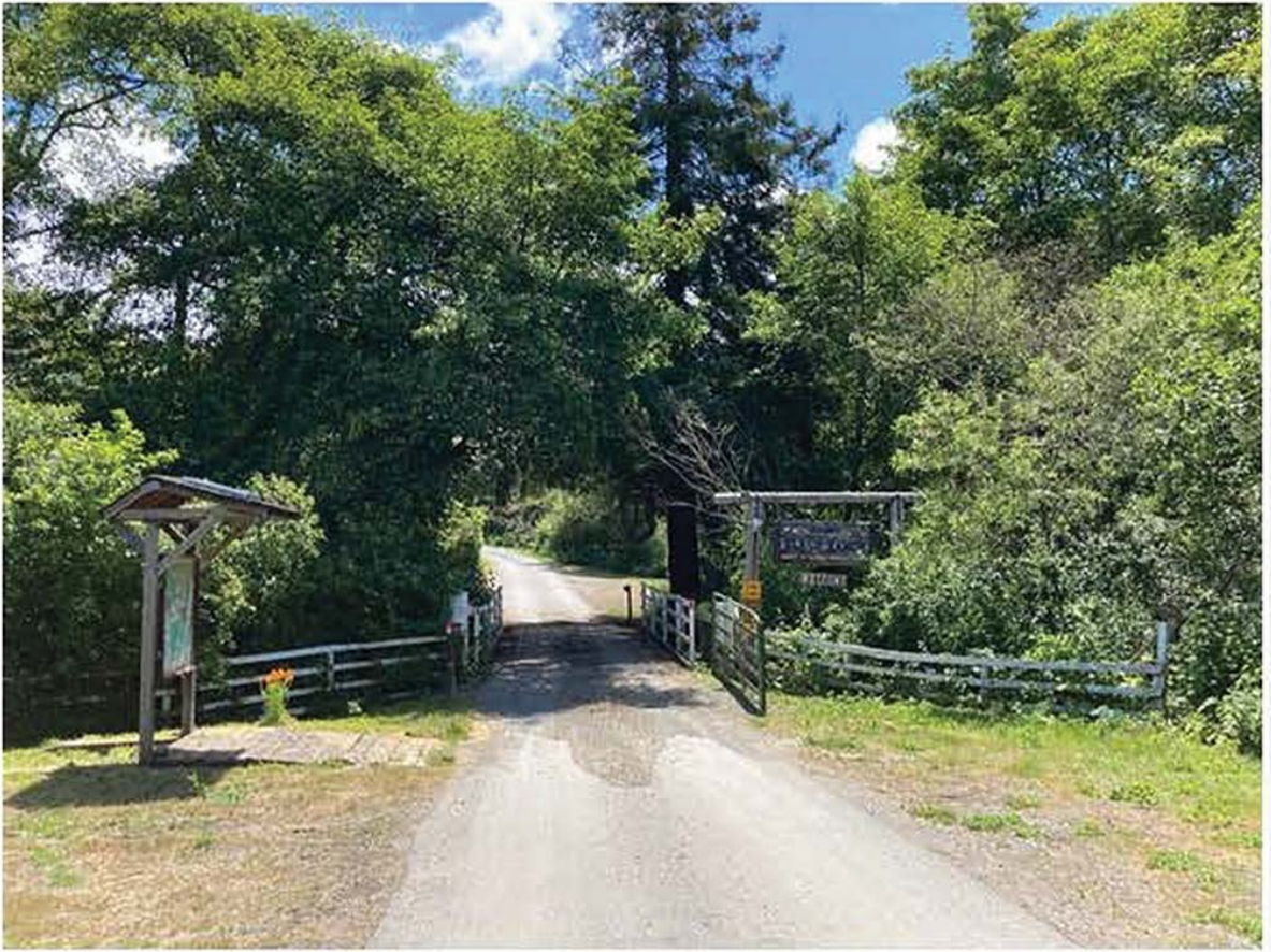
Elkus Ranch entrance when the bridge was intact in 2022.
