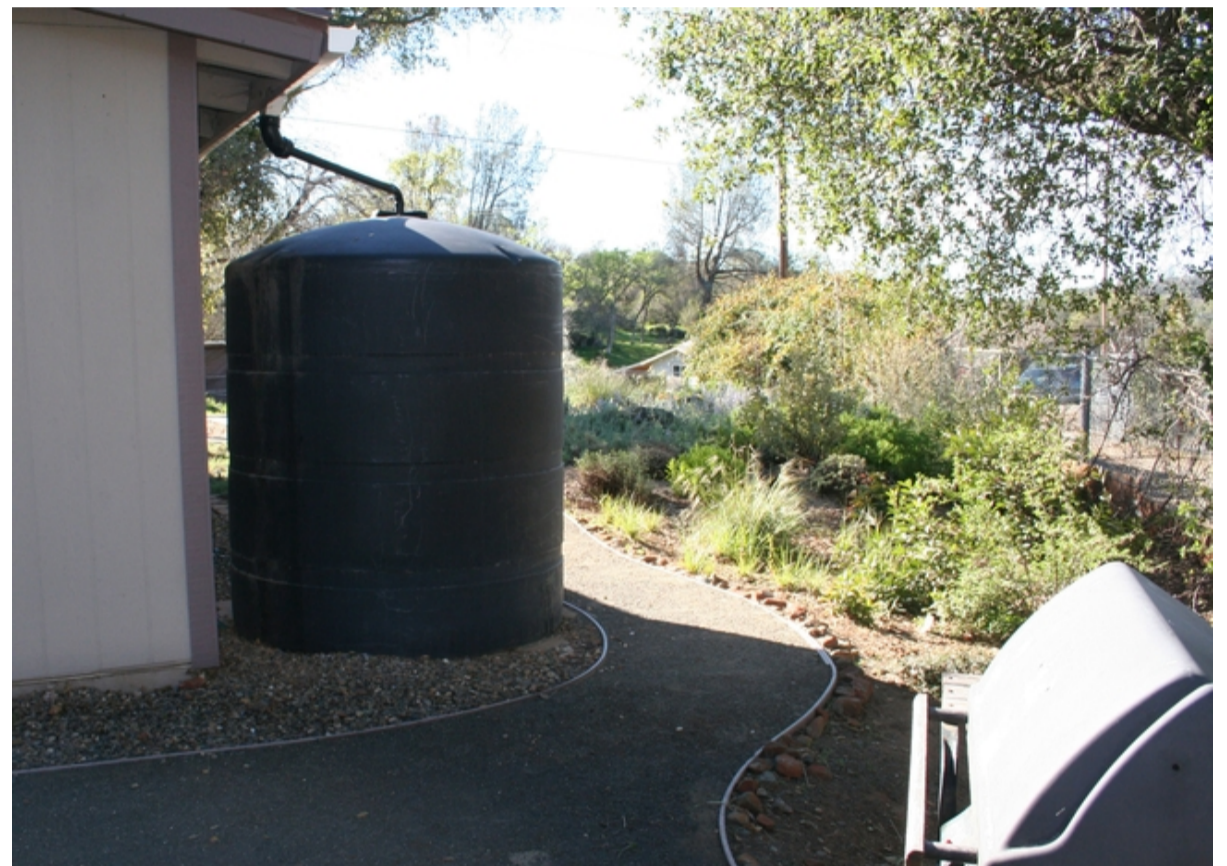
A foothill dwelling landscaped with a five-foot non-combustible zone. The building is also equipped with an extra large rain barrel that collects water during storms for irrigating plants.
