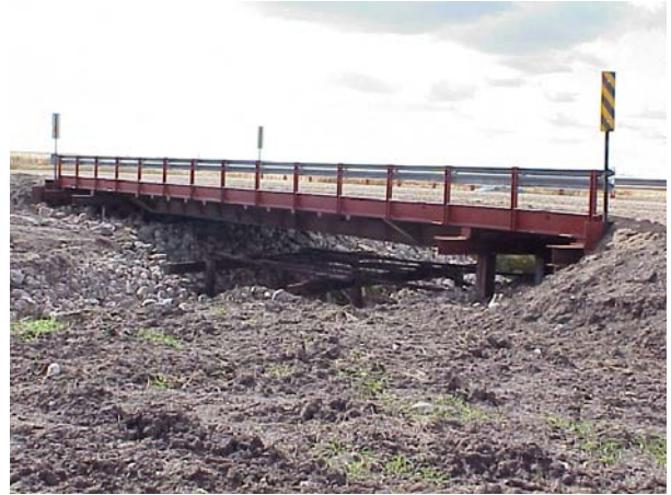
(b) Winnebago County Bridge
