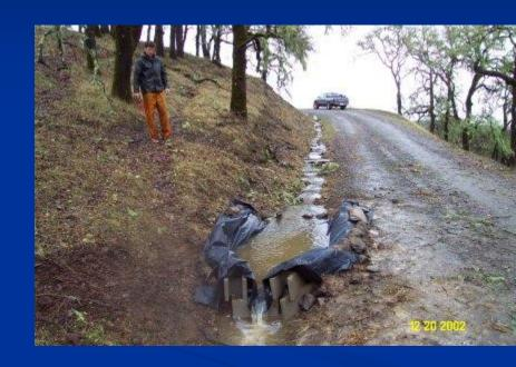
Cross drains are culverts or rolling dips that intercept and "relieve" ditch flow. They may be inadequately sized or spaced. As a result, ditches may erode or excessive runoff may be diverted down the road, causing rills and gullies.
