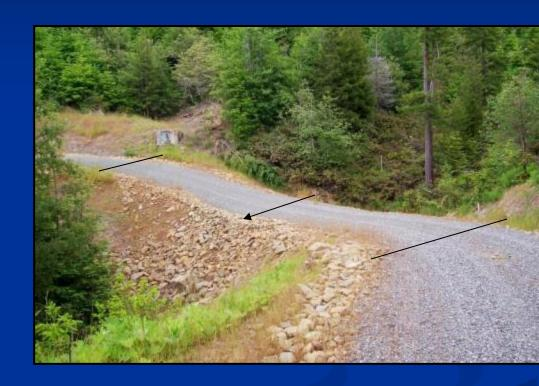
Sufficiently sized stream crossing is placed at "B". "C" is critical dip axis. "A" and "D" are cross drains placed to intercept road runoff and disperse it over land instead of into the stream.
