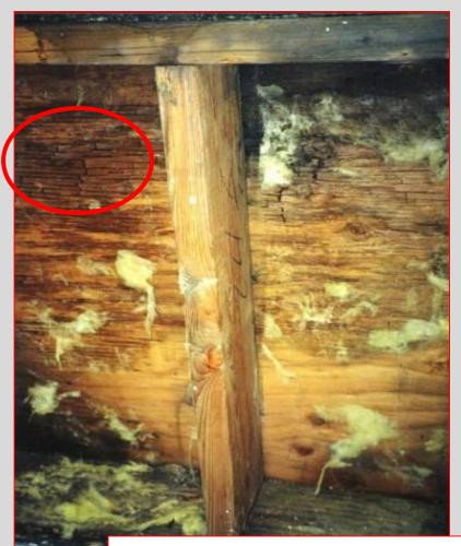
Leak at a window, with advanced decay in plywood sheathing. Some brown rot fungi have developed a specialized waterconducting hyphal mass called a "rhizomorph." A leak is no longer necessary. Water (usually from soil) can be conducted through the rhizomorph to the wood in your home. *Meruliporia incrassata* ("poria") is the most common "water conducting" fungus in North America, and the one most commonly found in buildings.
