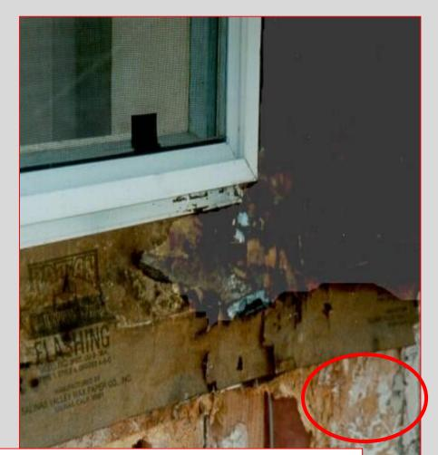
Leak at a window, with advanced decay in Oriented Strand Board (OSB) sheathing.
