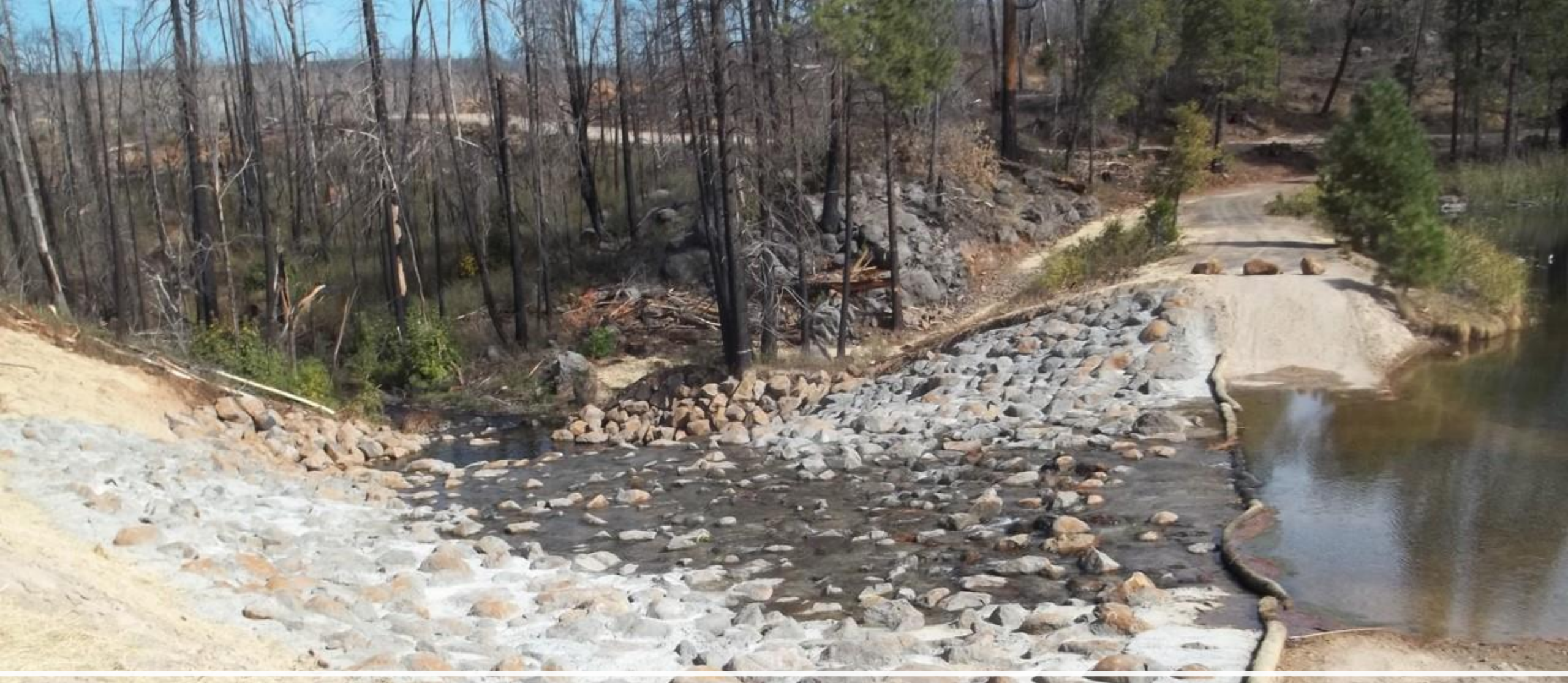
Final Spillway Repair- Grouted Rock Chute, 10/2015
