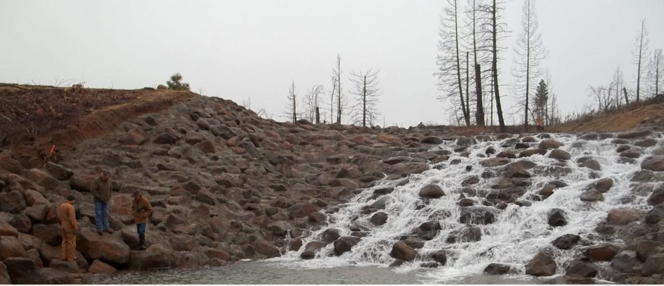
Final Spillway Repair- Grouted Rock Chute, 1/2016
