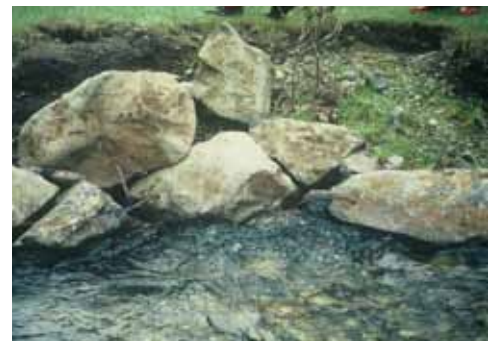
In-stream projects add rip-rap and other structures to support fish and prevent sedimentation.
