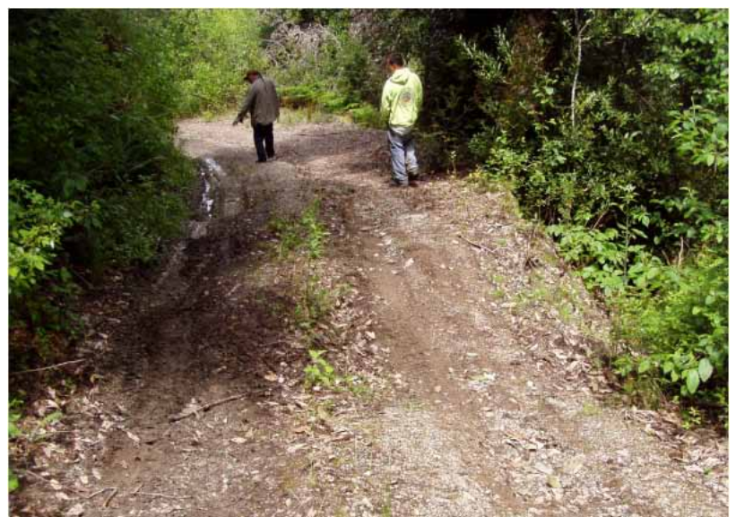
Road assessment and rehabilitation.
